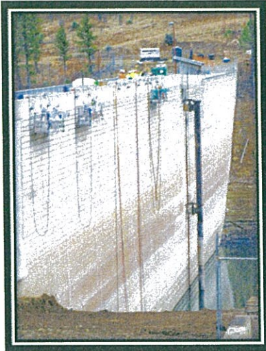
Grindstone Liner Installation
