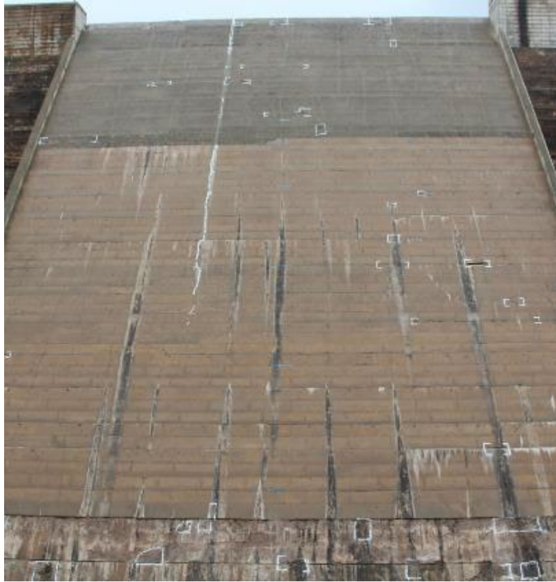
Photo 2: Grindstone Canyon Dam Spillway (October 5, 2022)
