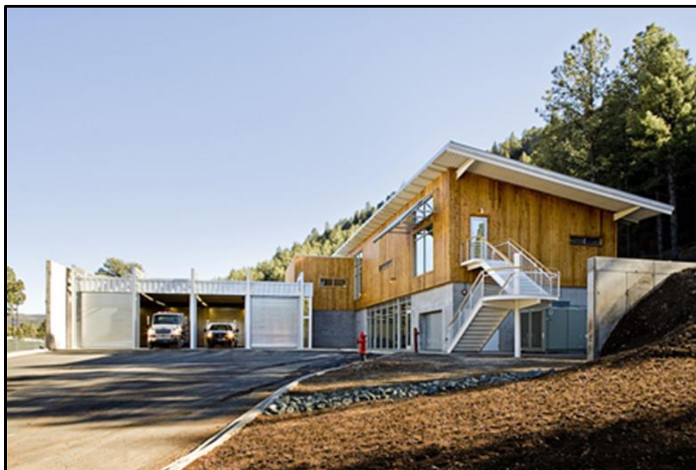
Figure 5-30: Village of Ruidoso Fire Department, Station 1.
